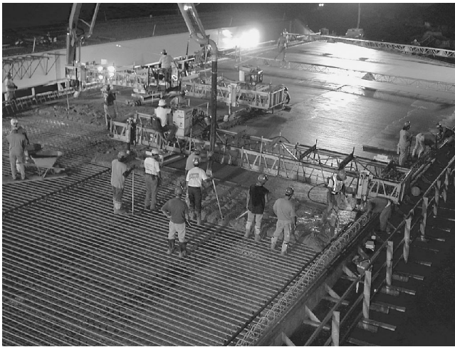
FIGURE 4 Twelve-hour concrete deck pour.
