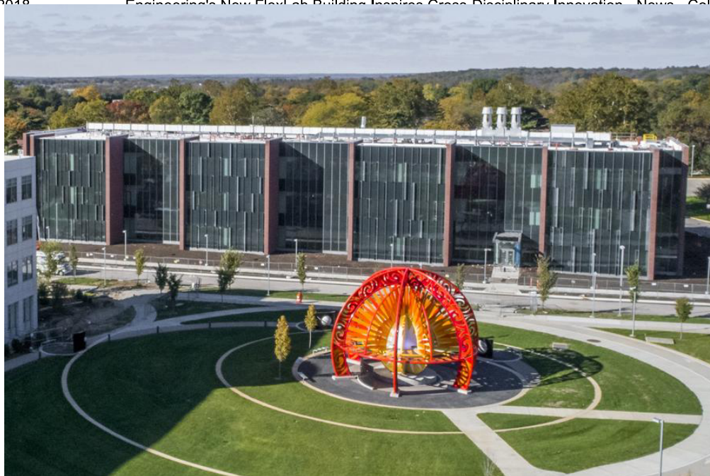
The new FlexLab building near the Voss statue in Discovery Park.
