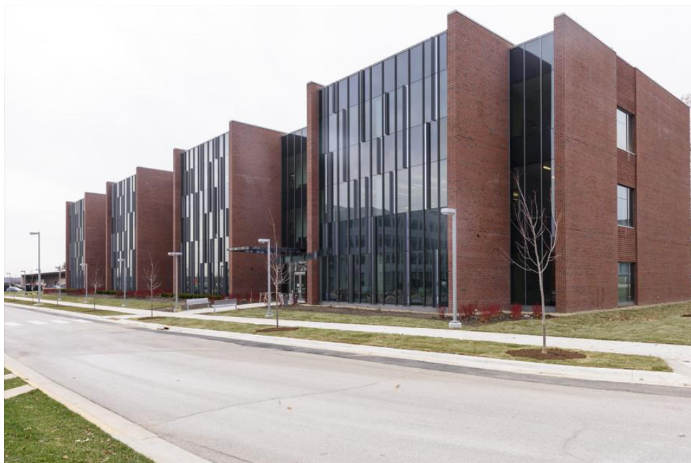
The new FlexLab building.
