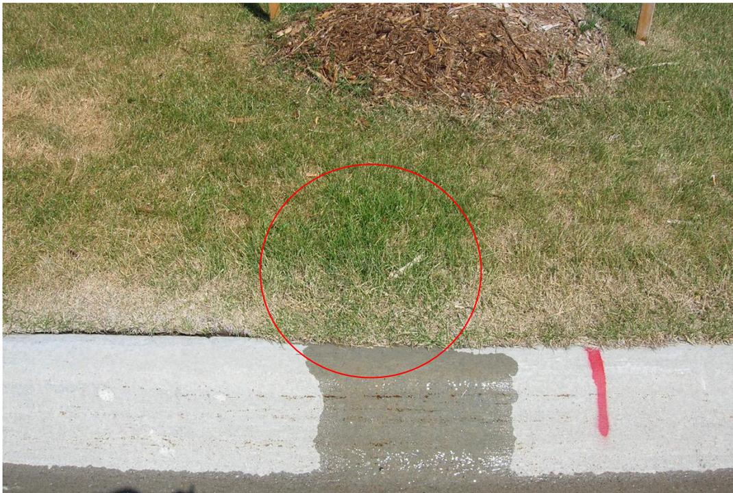
*Figure 5. Example of a buried sprinkler head.*
