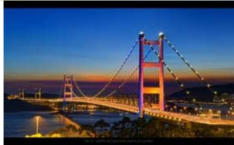
Tsing Ma Bridge in Hong Kong (approx. $20 million for 1000+ channels of data acquisition)
