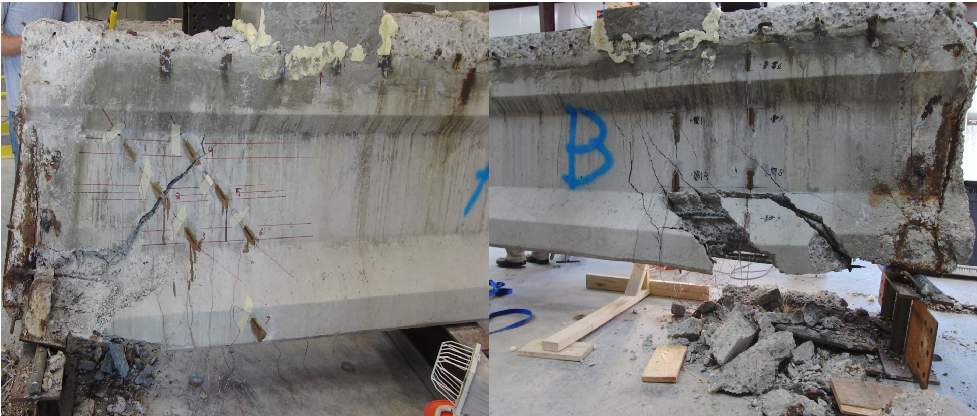
Web Shear Failure
